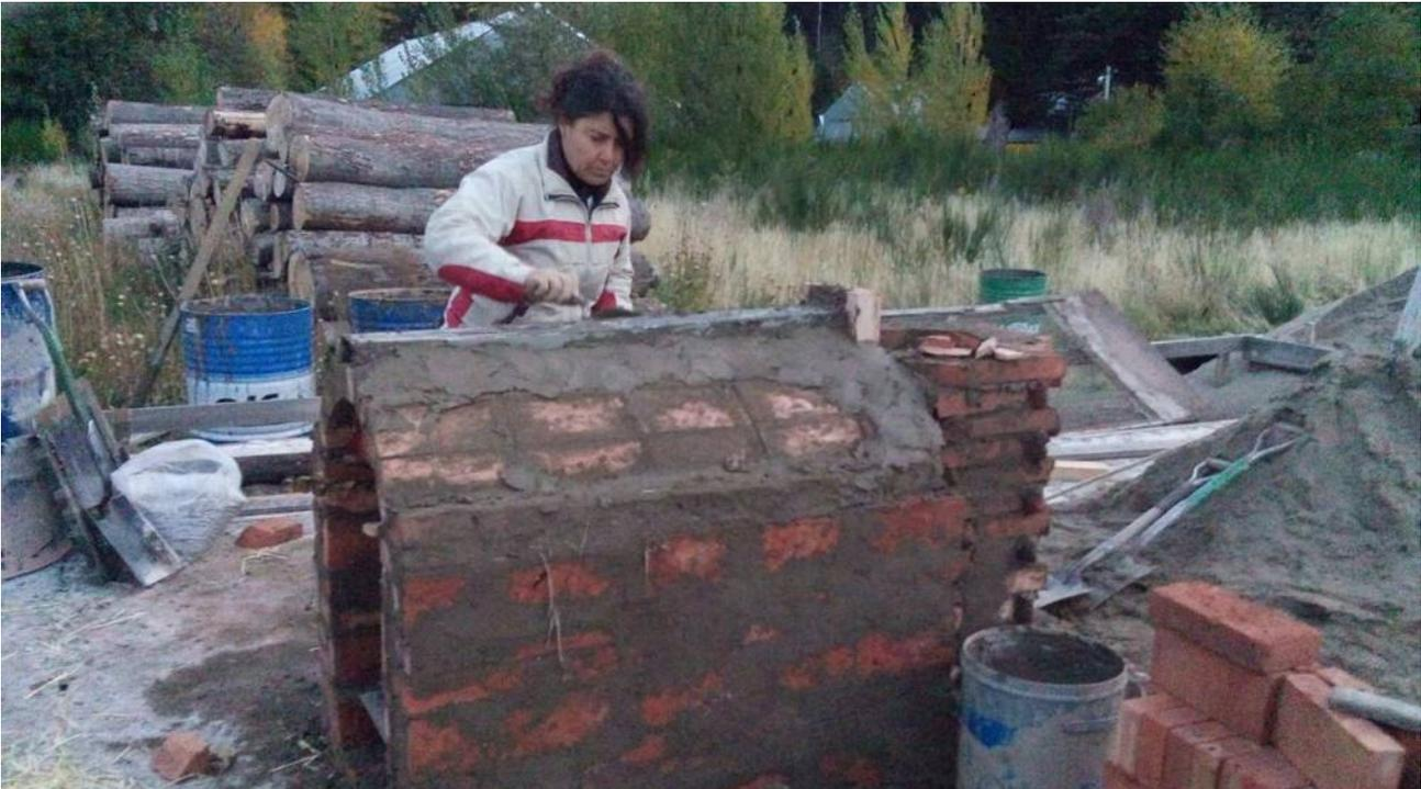
*Picture 8: End of day 1 build. Firebox and early courses of heat riser. P channel horizontal metal piece in place. We used a portion of a 200l drum as a cimbra (temporary support for the vault)*
